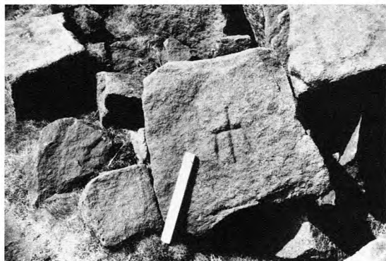
Plate 20 Mason's trident mark on a block of millstone grit on Hathersage Moor (at about SK 251807).
