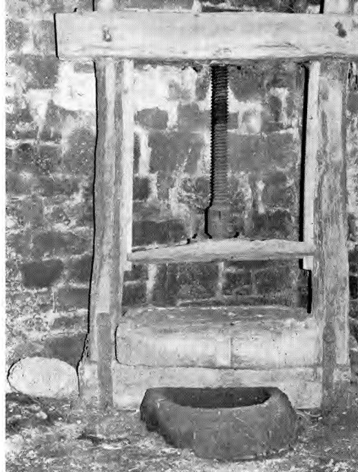
Page 323 (right) Cider-press at a cottage in Lone Lane, Penallt, showing the timber frame, screw press mechanism, press-stone and receptacle. The press board itself is missing; (below) the major part of a corn-mill-stone now used as part of a garden ornament at 'The Generals', Penallt. The near-radial grooves, although largely worn and weathered away, can still be seen clearly See D. G. Tucker, 'Millstone Making', pp 229-39
