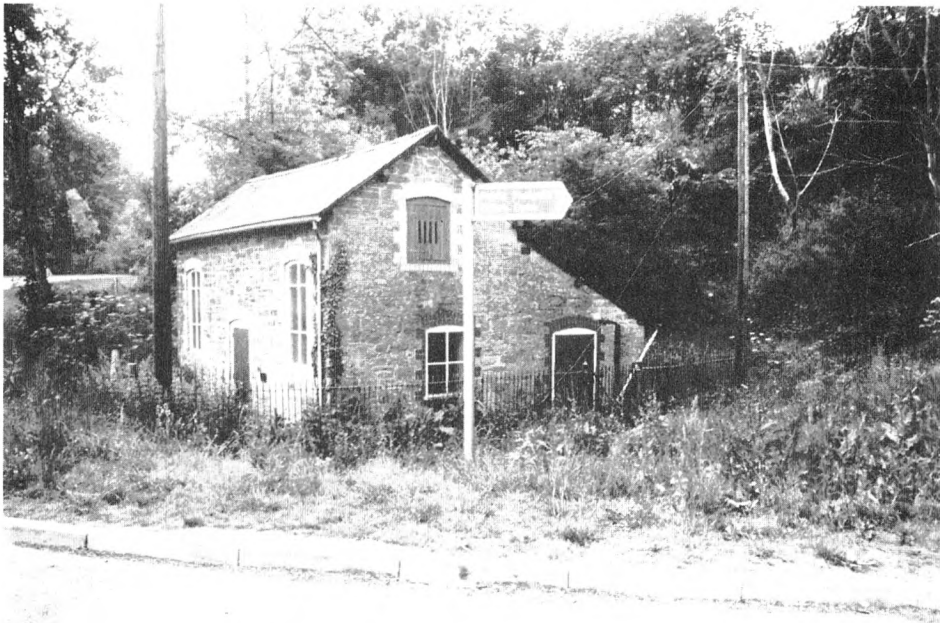
CROOKED WELL PUMPHOUSE
