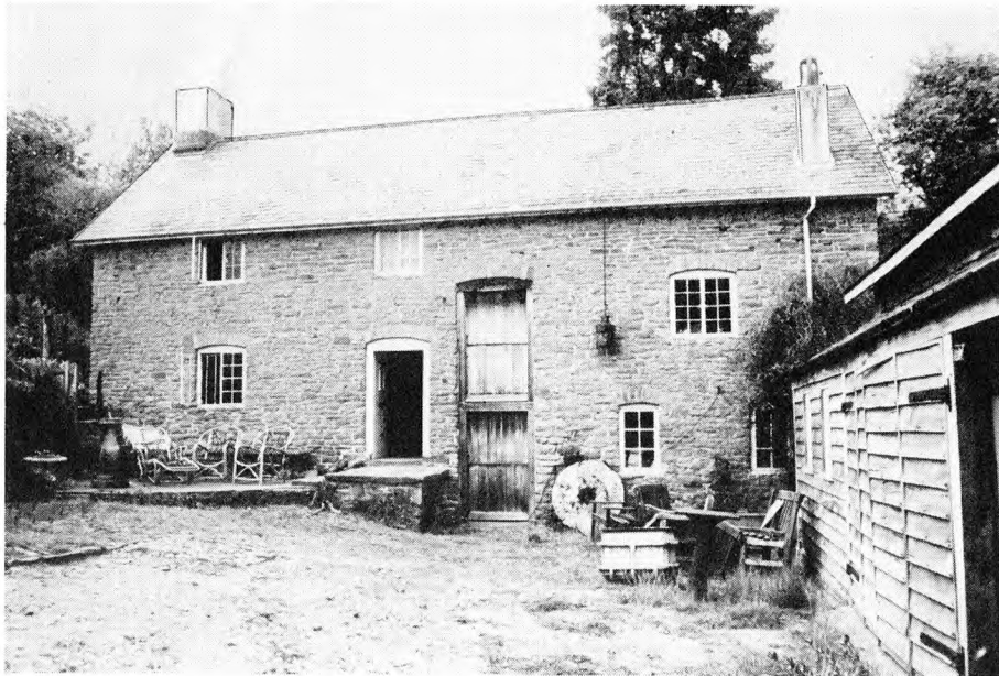
PLATE 3. Norton Mill (no.7). The water wheel is at the back; the mill is the right-hand part of the building.
