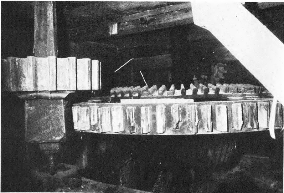
PLATE 4. The great spur wheel at Norton Mill, showing the bevel carried on it to drive a horizontal layshaft.
