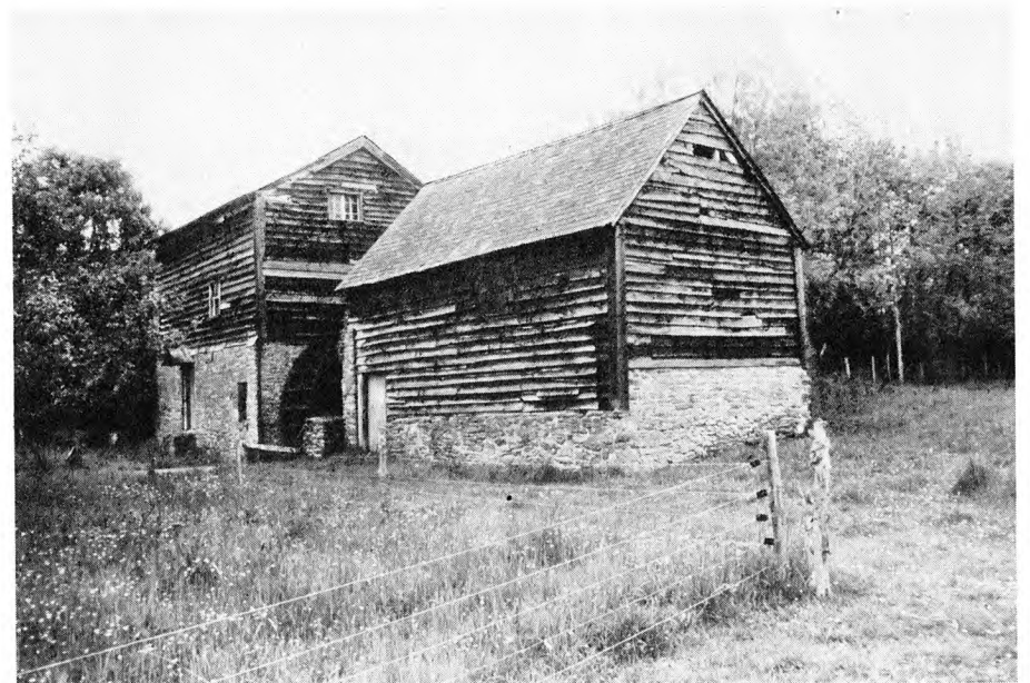
PLATE 5. Wegnall Mill (no.16). The mill is the building on the left, and the wheel can be seen between the mill and the barn.
