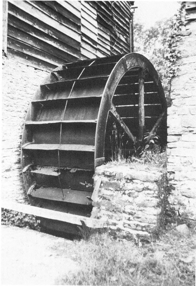
PLATE 7. The undershot water wheel at Wegnall Mill.
