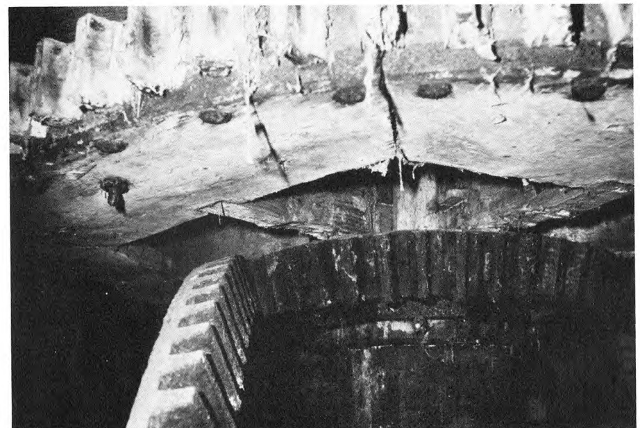
PLATE 6. Showing the construction of the wooden compass-arm spur wheel at Wegnall Mill, with the wallower and pit wheel showing below.
