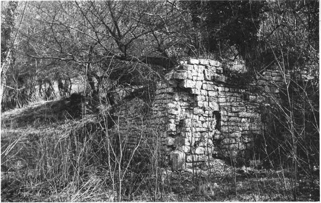
Pond No. 25 (Upper Mill)
