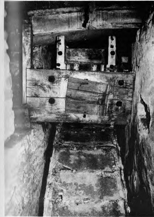
Plate 45. Tugford Mill (e/7). The internal wheel and header box.
