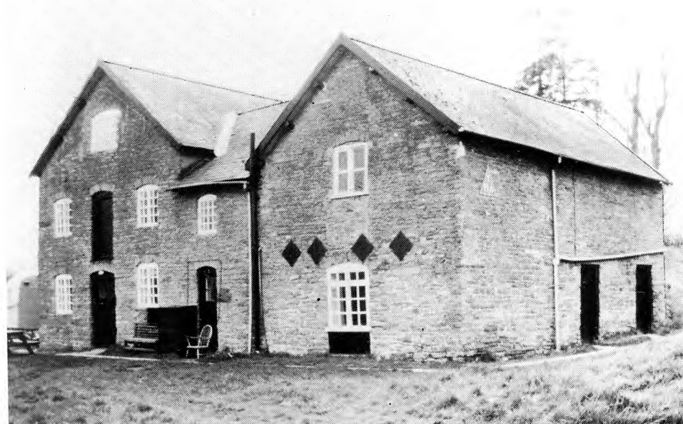
Plate 29. Clun Mill (c/15), which has served as a youth hostel for over fifty years. The mill itself was the left-hand part of the building.
