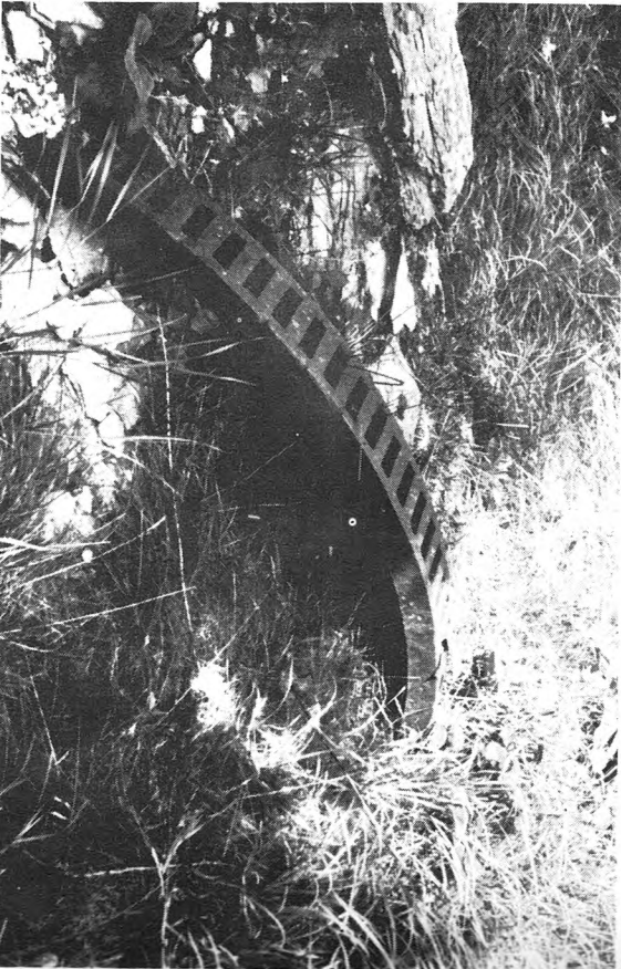
Iron Factory (D/14). Above: the cottages; mill ruins at end. Below: piece of gear wheel with mortices for wooden teeth.
