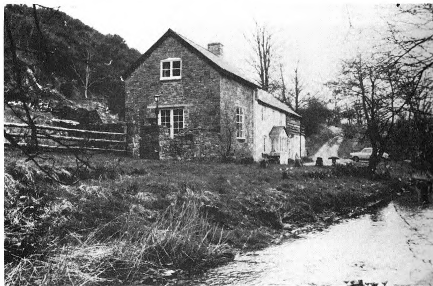
Bettws Mill (B/7), now a residence. River Edw in foreground.
