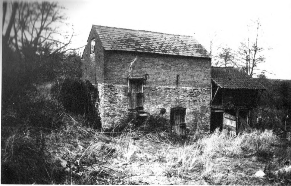
Bage Mill , in parish of Madley (No 120), showing brick upper parts on stone-built base, suggesting an early extension or rebuilding.
