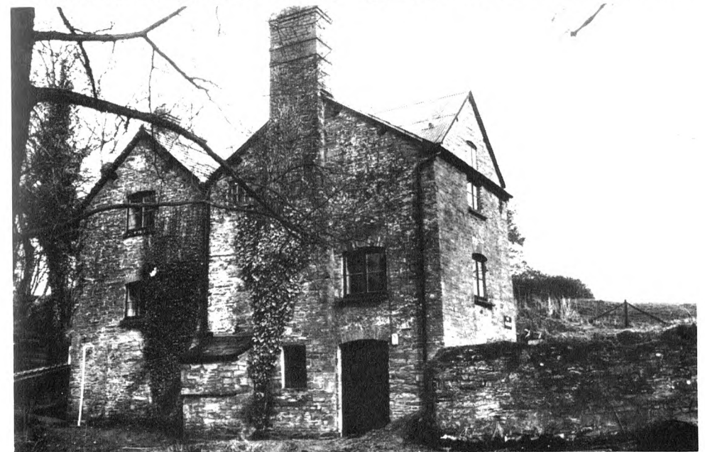
Whitney Mill (No 138) . A corner of the wheel-pit is just visible on the far left-hand side.
