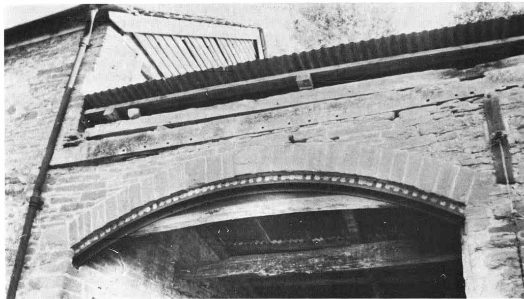
Arch supported on segment of gear at Dorstone Mill (number 32)
