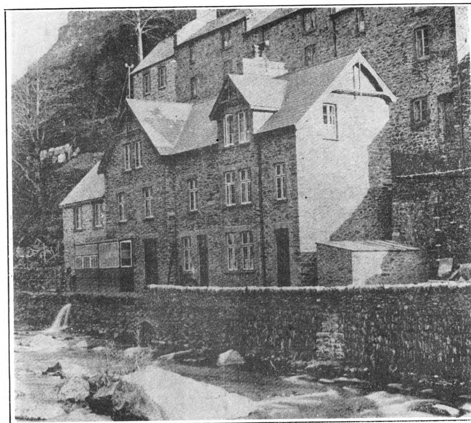
Plate 9. The hydroelectric generating station at Lynmouth, Devon. (From "Electrical Engineer", 1899.) This was opened in March 1890, and within a few years was using a pumped-storage system with a head of 760ft. and a reservoir capacity of nearly 200,000 gallons to help with peak loads. The power came from the East Lyn river, and about 75KW could be generated directly, with another 75KW when required from the water pumped to the high reservoir at times of low load. The station remained in use until destroyed by the great floods of 1952. By this time it had internal combustion engines to supplement the water power. (See Section 2 of article)
