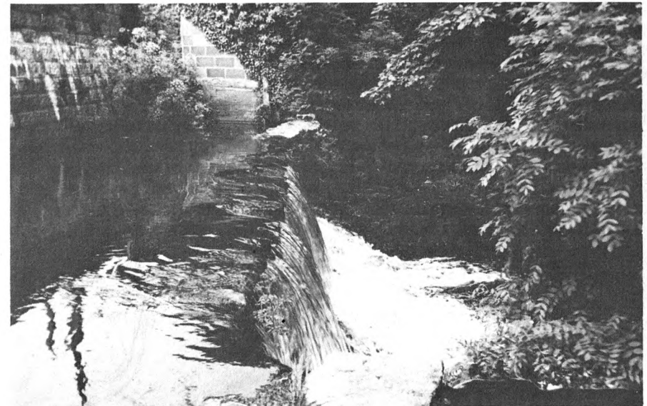
Plate A Present-day view of the weir on the East Okement River which formerly provided the head for the Okehampton hydroelectric station. (Photo by D.G. Tucker)
