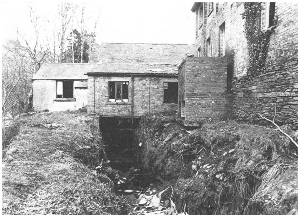
Plate 3 The building of the Keswick electricity-generating station from the tail-race. The extension which housed the Gunther turbine is on the left. The building on the right played no part in electricity generation, and was used for the manufacture of soya flour during World War II. (Photo by D. G. Tucker)
