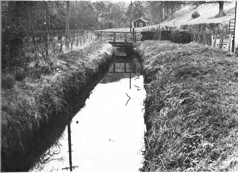
Plate 5 The head-race at the Keswick generating station (Photo by D. G. Tucker)
