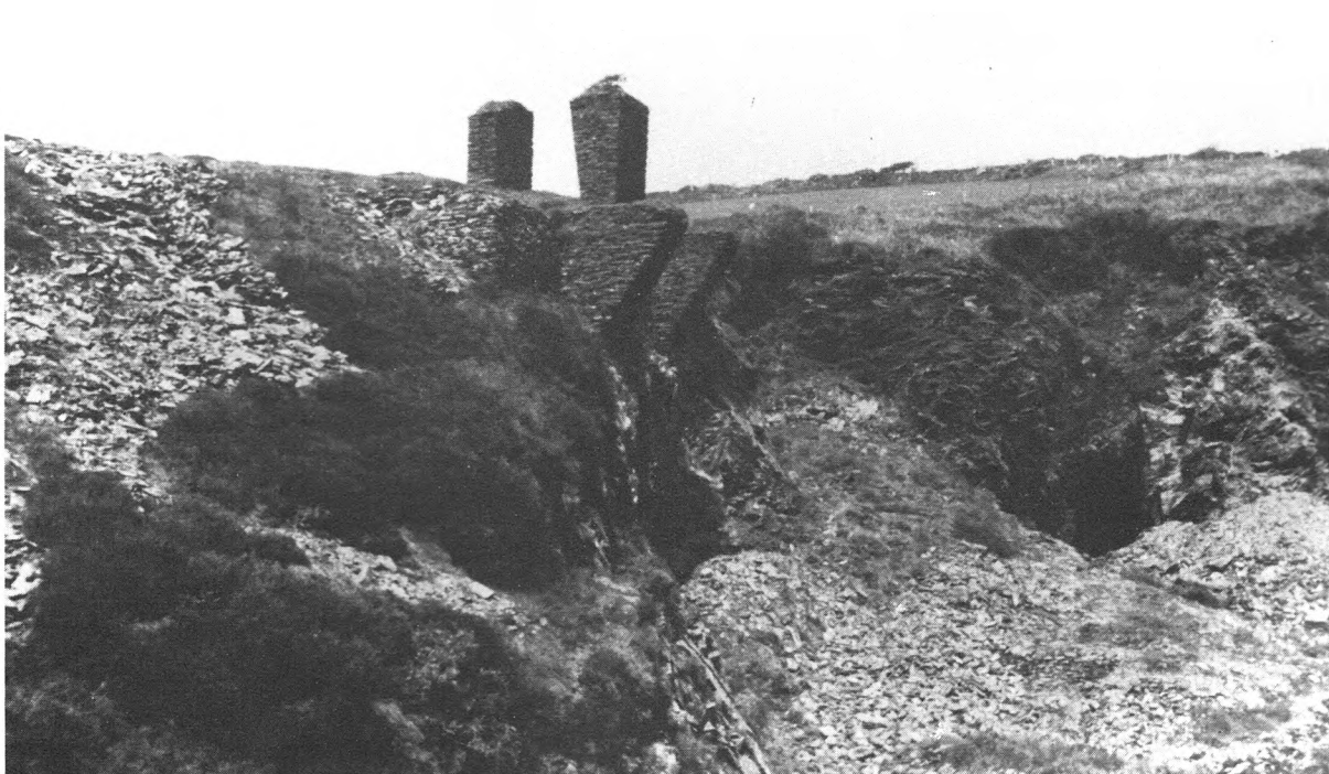
Plate 6 Part of Summerton Quarry (No. 52) looking northwards, showing the stone piers on the western lip of the quarry (centre) and the western mine entrance or 'cave' (right).
