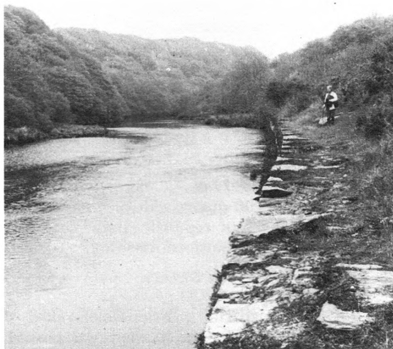
Plate 4 The old slate quay at the Forest Quarries (Nos. 39-44) on the river Teifi, viewed up-stream.
