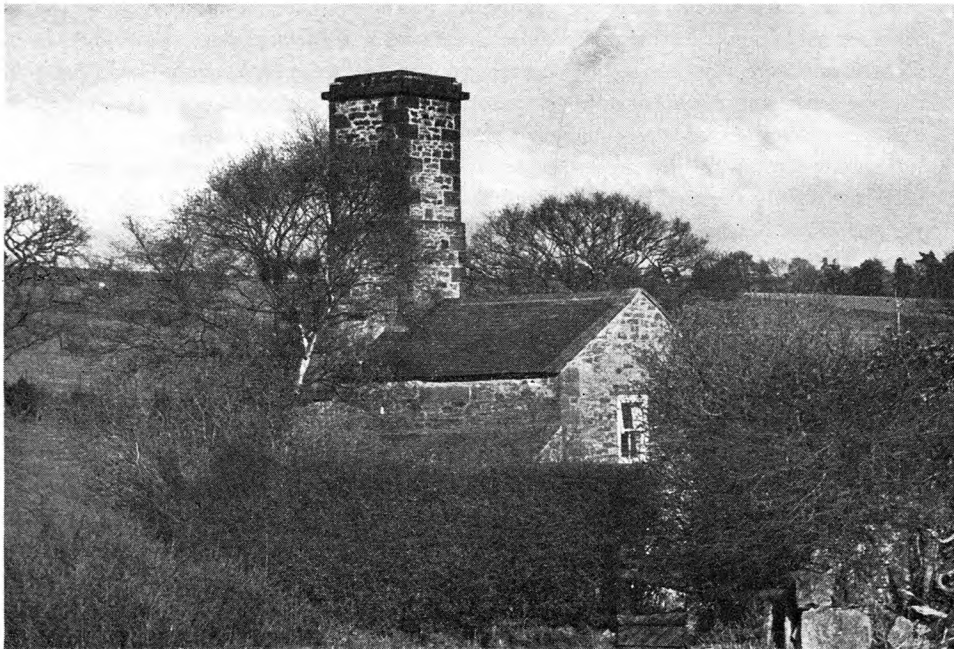
Above: The Langley smelt-mill in Northumberland, about 8 miles west of Hexham, was built in 1768 by the Greenwich Hospital Commissioners to smelt ore received as royalties from the London Lead Company who were their lessees in important lead-mining areas in the north, especially on Alston Moor. Much experimental work was carried out at Langley, and it was an advanced mill for its time. In particular, efforts were made to obviate the poisoning of the animal life and vegetation of the area, and eventually a flue, three-quarters of a mile long, was built to this rather unusual chimney high up on the moor at Stublick (grid reference NY 841 611).
