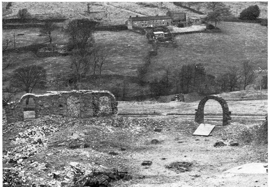
The Great Octagon Mill, Arkengarthdale, built about 1700, was one of the finest buildings associated with the lead industry. As can be seen from the illustration, little now remains of its former grandeur. (Grid reference NY 996 037).
