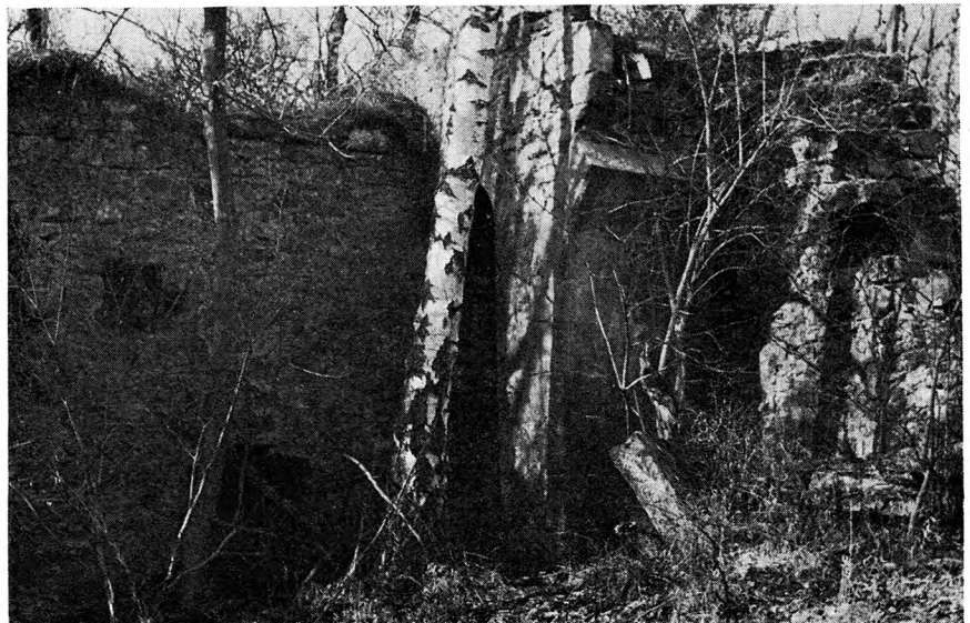
Right: Remains of the Fallowfield smelt mill showing an arch above the presumed site of an ore-hearth. This mill (grid-reference NY 937 675) was built about 1770, but there had been earlier smelters nearby.
