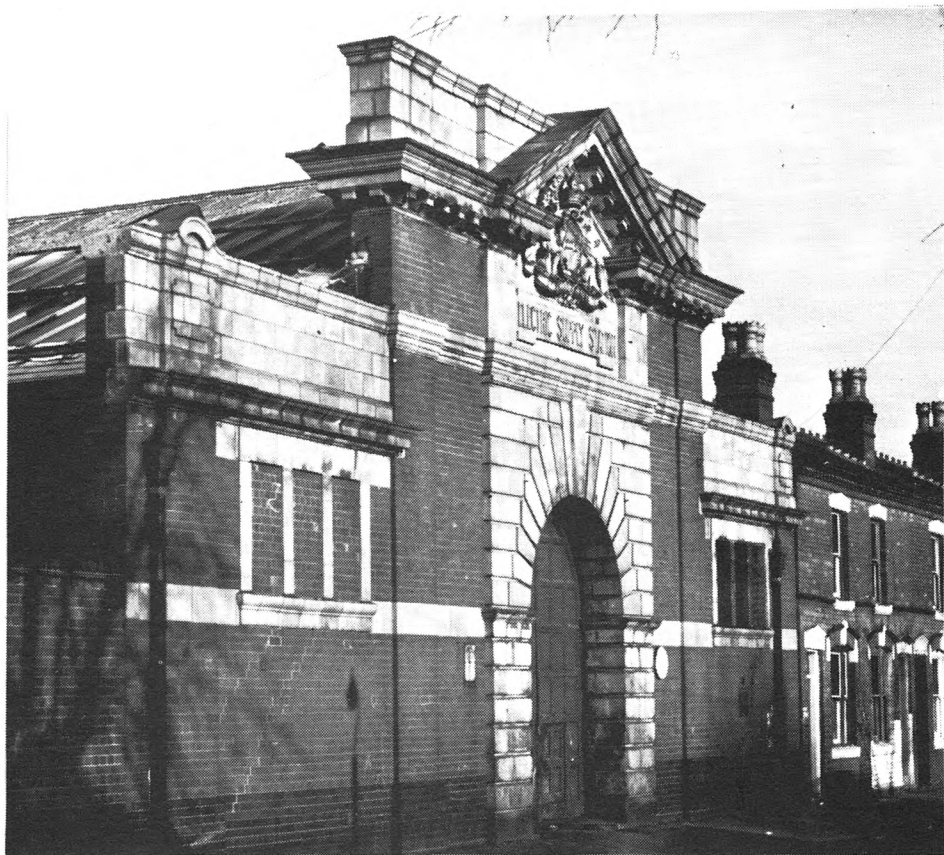
Sub-station at Court Road, Birmingham, 1906. SP 973 845.
