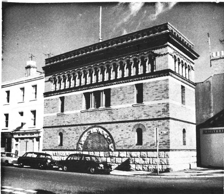
Photo 6. Sub-Station at Cheltenham, 1895. SO 948 225.
