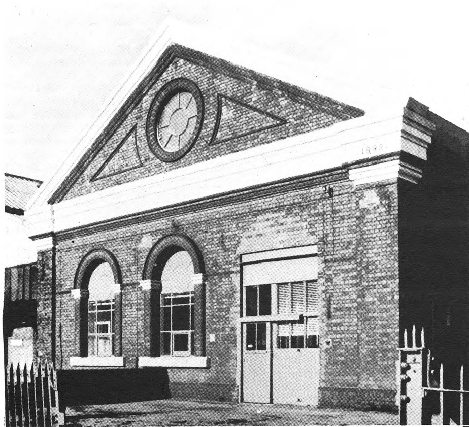
Photo 1. Facade of generating station of South Staffordshire Tramways Company, 1892. Pleck, near Walsall. SO 994 976.
