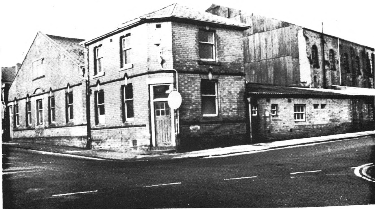
Photo 8. Redditch, 1898-9, with later extension. SP 043 673.
