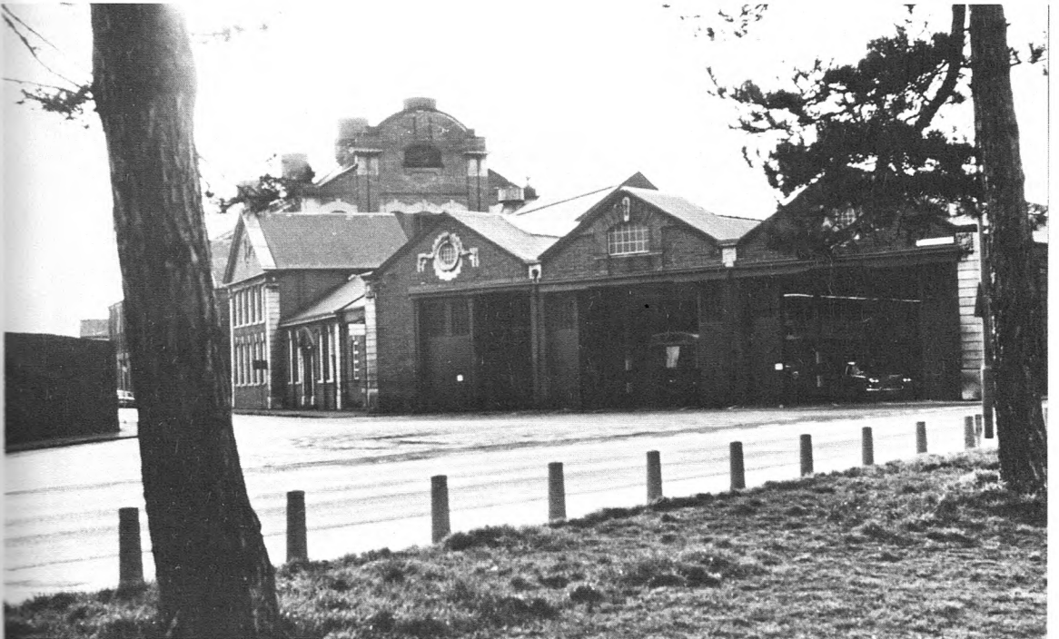
Plate 5 Ipswich generating station behind the offices of the old Electricity and Tramways Departments, with the old tram sheds in the foreground. With the refuse destructor, which stands well to the right of the tram sheds (see Plate 4), the whole made a very extensive municipal complex. Built 1903.
