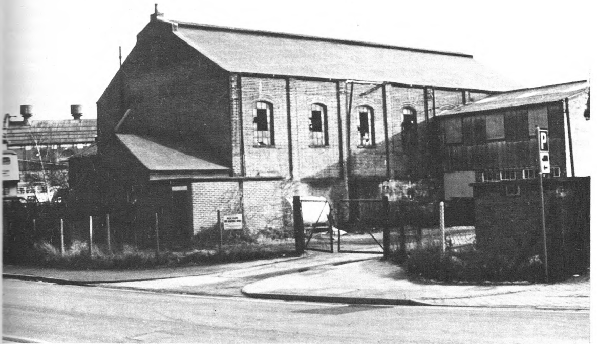
Plate 4 Refuse destructor at Ipswich. Steam was fed by an external steam pipe to the electricity generating station, seen behind on the left. Built 1903.
