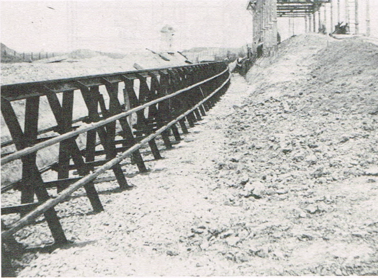
(a) photograph of track before conductor rails affixed. Courtesy of Gloucester Railway Carriage and Wagon Co. Ltd.,
